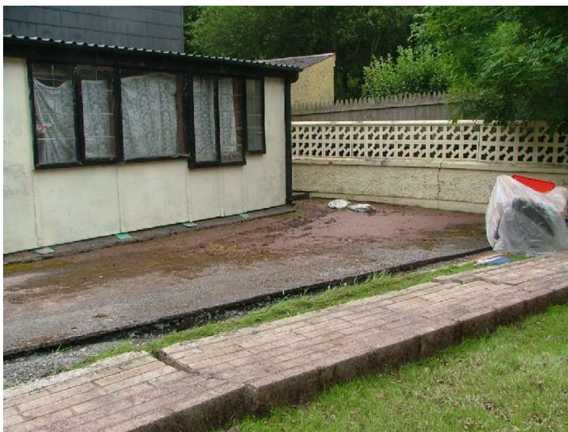
Residential Property – Behind Meeting Hall – Church Road – Wall Knocked
