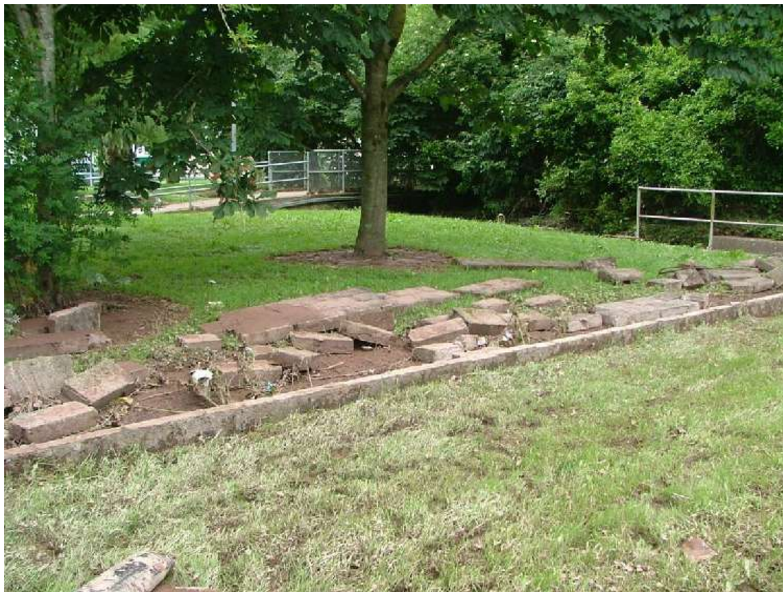
Meeting Hall - Church Road - Wall Knocked
