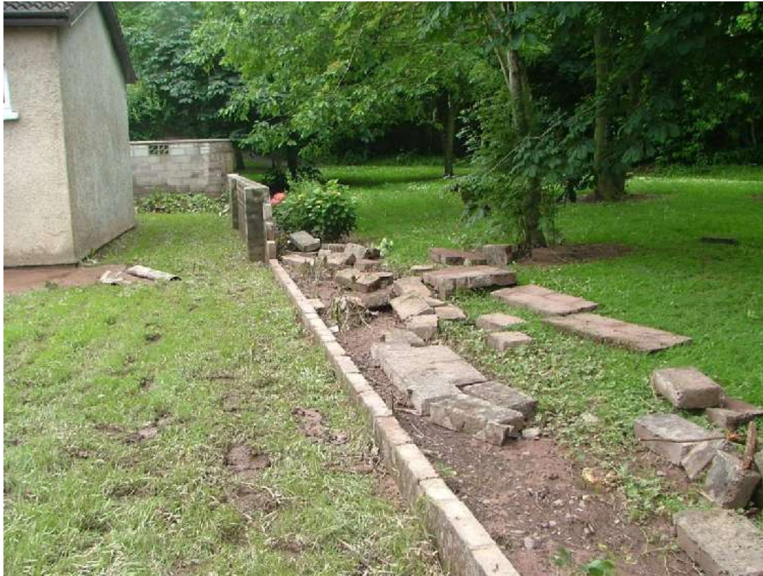
Meeting Hall - Church Road - Wall Knocked
