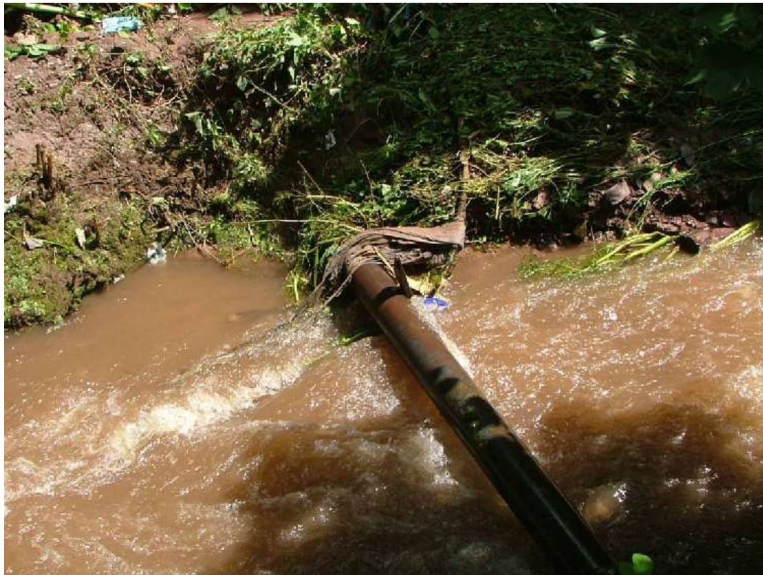
Donnybrook River – in Park – Pipe Crossing
